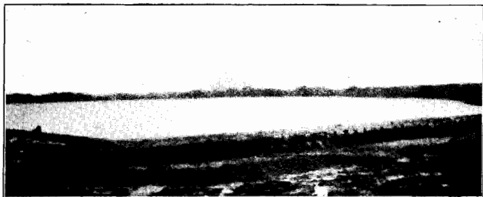
STORAGE RESERVOIR AT POTRERO — 2,500,000 BARRELS
