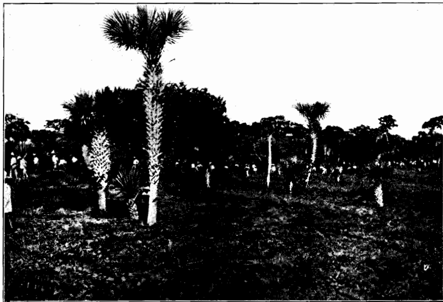
CLEARING JUNGLE FOR PETROLEUM CAMP
