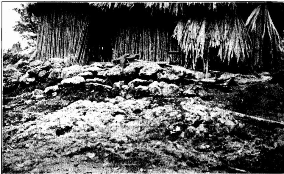
PEON HOUSES BEFORE OIL DEVELOPMENT BEGAN
