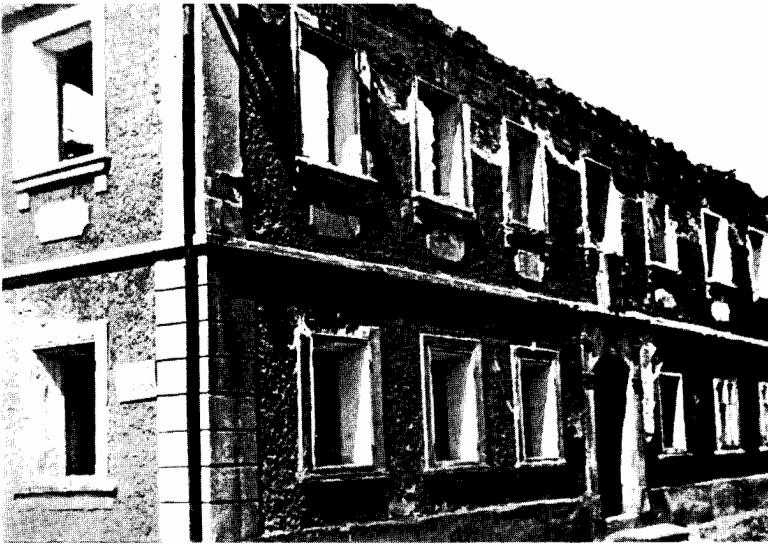
Derelict German School in Eger-Karlsbad District.
