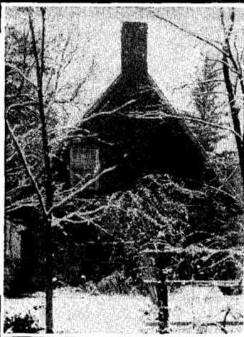
Below: Front of the Tappan Shrine, showing, left, a frame structure erected subsequent to the Revolution. The window in the roof to left of the tree opens from the room which was occupied by Washington.
