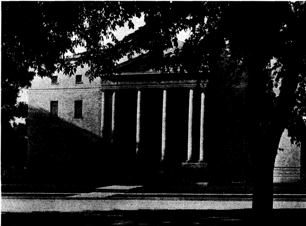
Masonic Temple, Fort Collins, Colorado.
